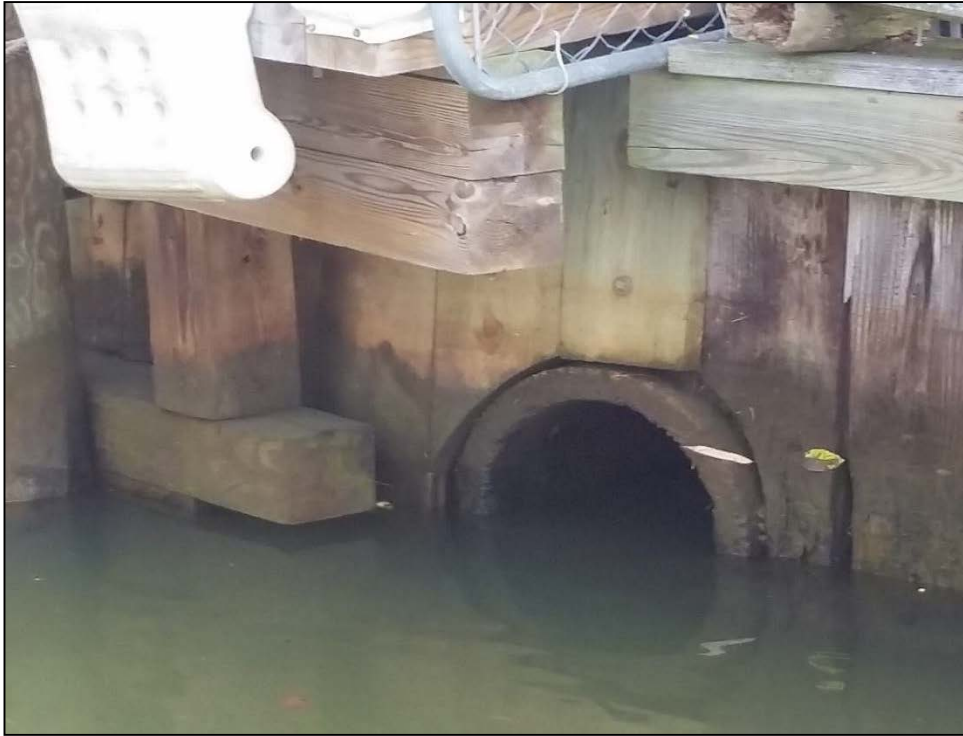
Stormwater outfall discharge to the canal.
