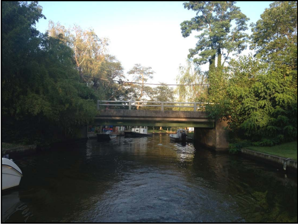
Low bridges restrict access by large boats for much of the canal.
