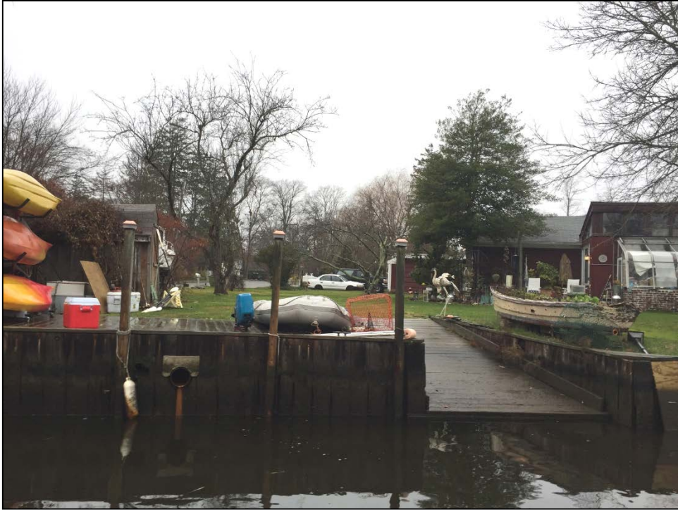
Stormwater outfall discharge to the canal.
