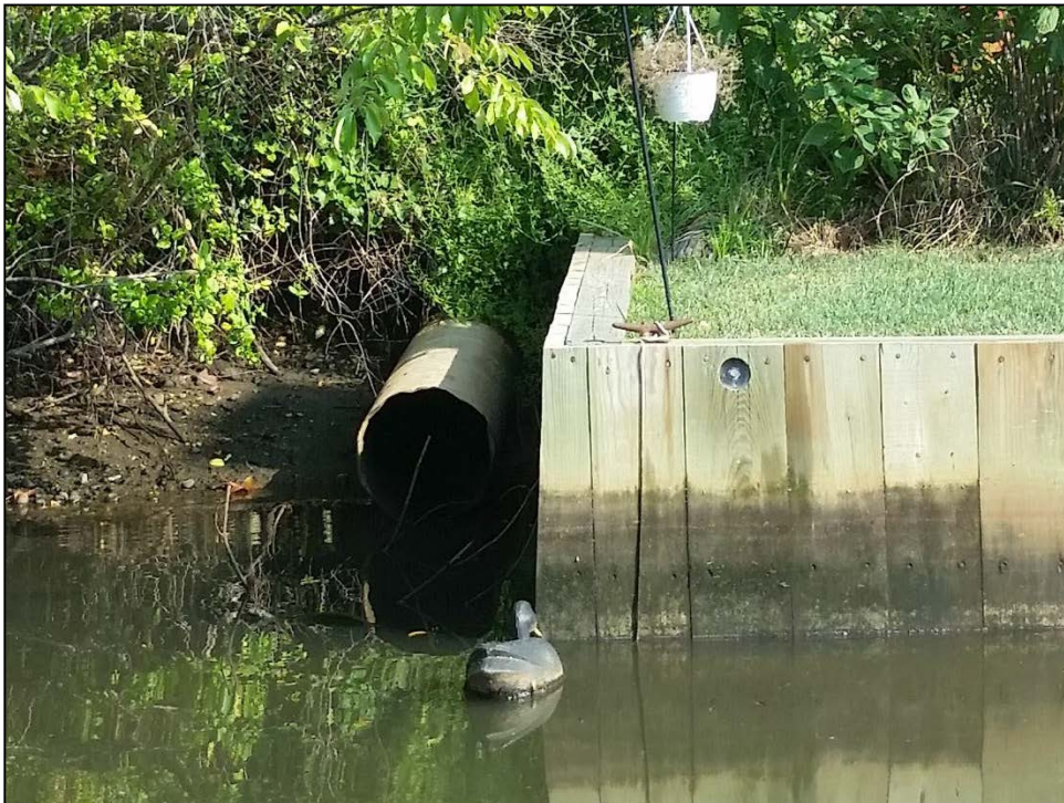
Stormwater outfall discharge to the canal.
