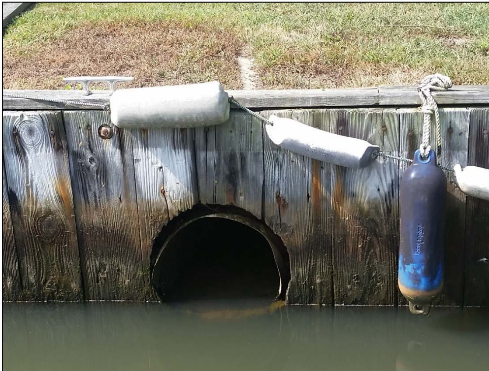
Stormwater outfall discharge to the canal.
